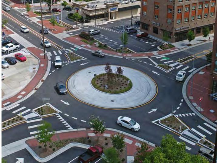
Roundabouts will deter speeding through intersections as vehicles will be forced to slow down to navigate the roundabout. Roundabouts do require a larger footprint to install and may be too large to incorporate into the road ROW on Peninsula Road. Collisions increase at roundabouts as those drivers no familiar with them, may have difficulty navigating through the roundabout.
